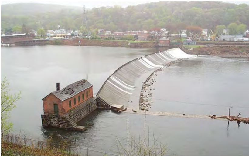
Figure 1. Example of a Dam acting as a barrier to anadromous fish passage. Photo taken on 4/28/2008 of Derby Dam in Shelton, CT; photo credit CTDEP/Inland Fisheries Division.
