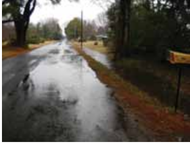
Station Road, Facing Northeast
