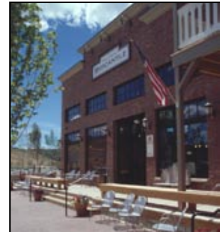
Case Study: Built in the first phase of the Hidden Springs, this post office/general store/ice cream parlor faces the village green, which functions as a community gathering place and backdrop for seasonal events.
