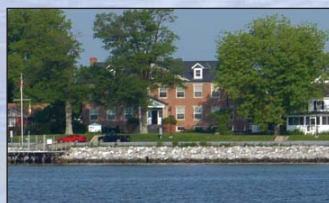
The main administration building at the UMCES Chesapeake Biological Laboratory.
